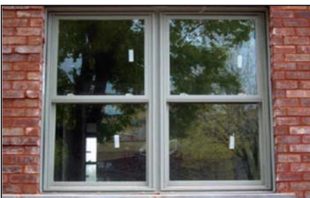
Figure 7 – New fibreglass windows
