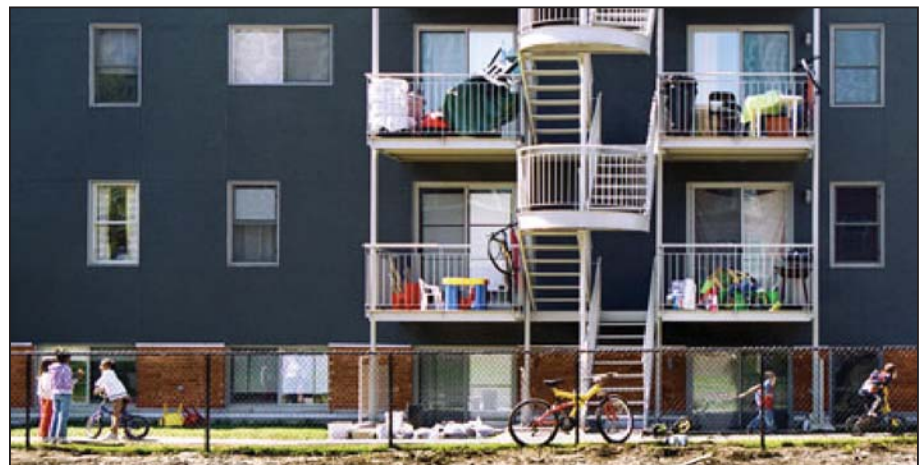
Figure 8 – New patio doors and balconies
