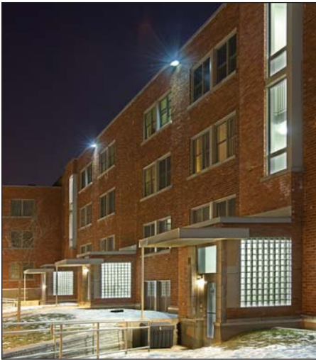
Figure 3 – Glass block reused in new entrances
