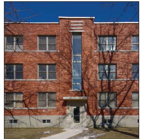
Figure 11 – View of renovated building
